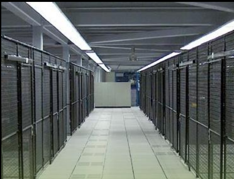
Old Open Inefficient Design
