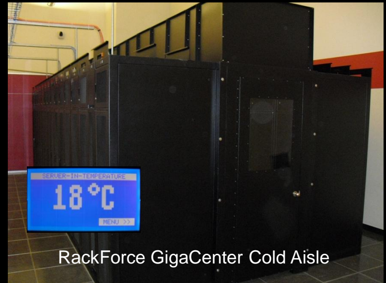
New Enclosed Cold Aisle Design
